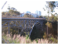
1 st Avenue Bridge
